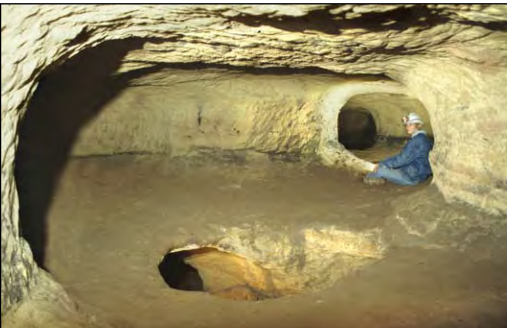
Plate 3 (bottom left). A step in the floor profile between the two levels in Rouse's mine has been fashioned into a trough just over the rock lip, which may have been a manger for the mine ponies. The brickwork is part of the air raid shelter modifications.
